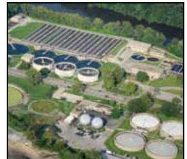
Water treatment facilities utilize SmartSonic.
